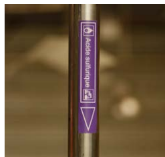
Pipes identification
